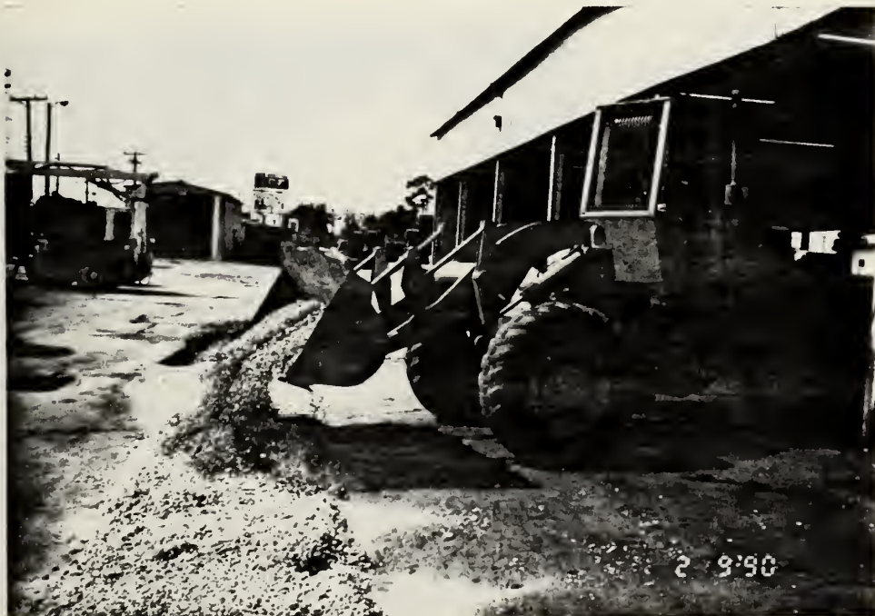
Figure 2.4 Front End Loader Placing Coarse Aggregate
